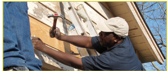
Volunteers engage in renovation efforts
