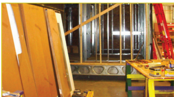
Building dormitories takes place inside FPCC's construction space
